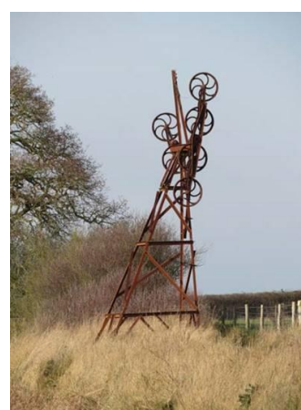
Ballast barge jetty and bucket chain pylon gravel conveyor system, Alresford Creek
