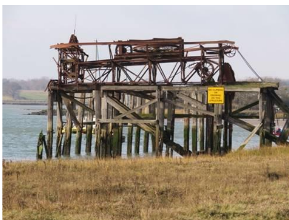
Ballast barge jetty and bucket chain pylon gravel conveyor system, Alresford Creek
